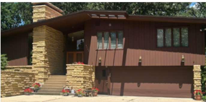
The Ray and Marian Sweeney home at 4306 Waite Circle. Built in 1960. Photo taken on June 26, 2024 by Tom Martinelli
